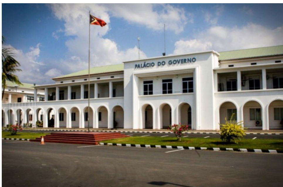
Picture 2 : Timor Leste Government Building 11
